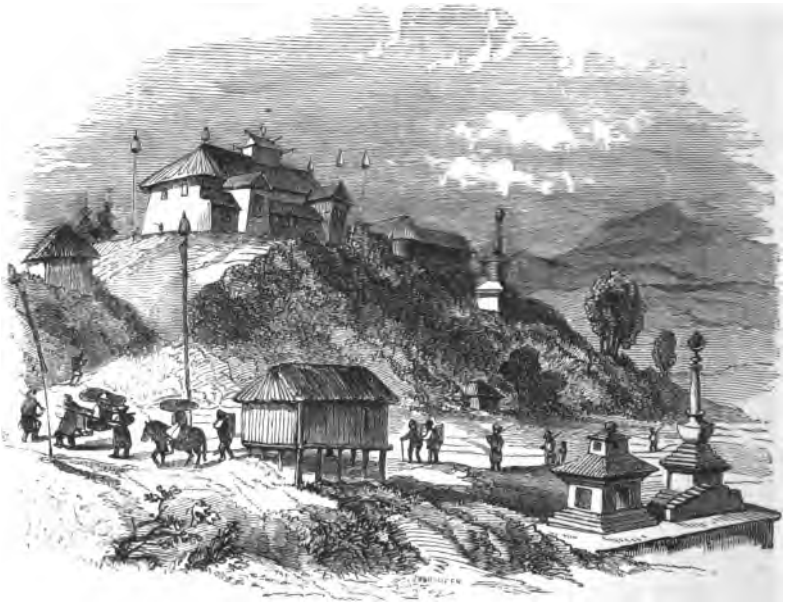
RAJAH'S RESIDENCE, AND THE HUT ASSIGNED TO US. ARRIVAL OF THE DEWAN.
