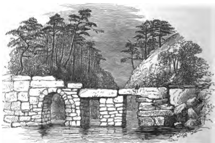
OLD BRIDGE AT AMWEE.
